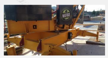
entire concrete slab was angled to facilitate heavy rainwater runoff. Entirely unsuitable for erecting and operating a crane.
